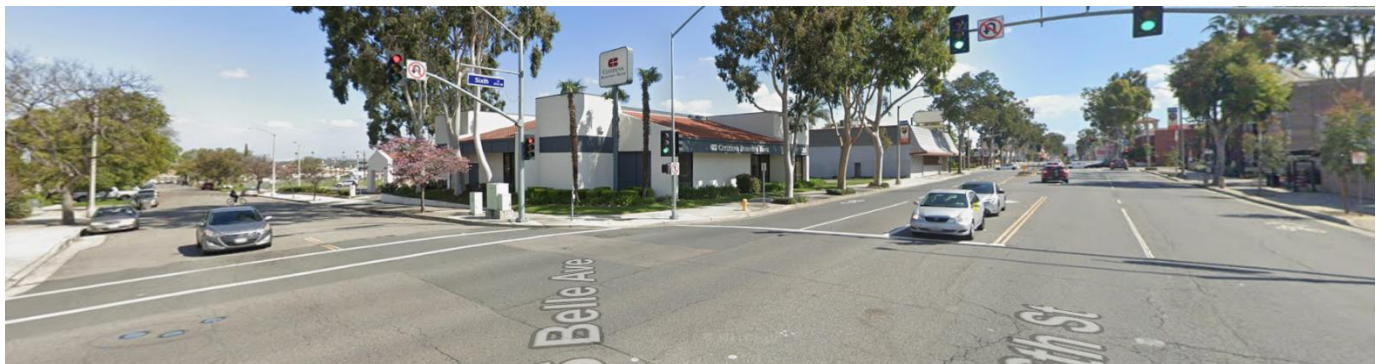
View Looking Northeast from W. 6 th St. and S. Belle Ave.
