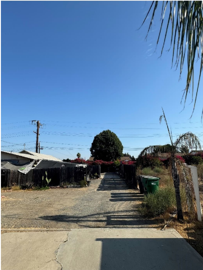
LOOKING S'LY IN THE FRONT OF THE PROPERTY
