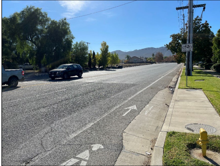
Figure 7. South Lincoln Avenue (view south; December 12, 2023).
