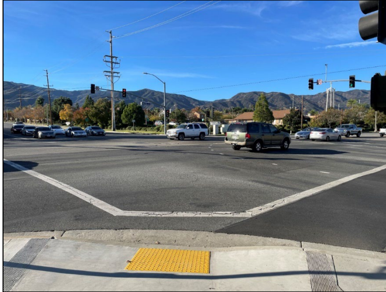
Figure 3. Project Area Overview (view southwest; December 6, 2023).
