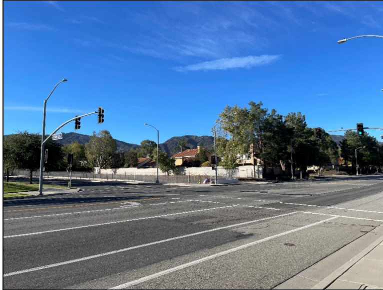
Figure 8. Oak Avenue (view southwest; December 12, 2023).
