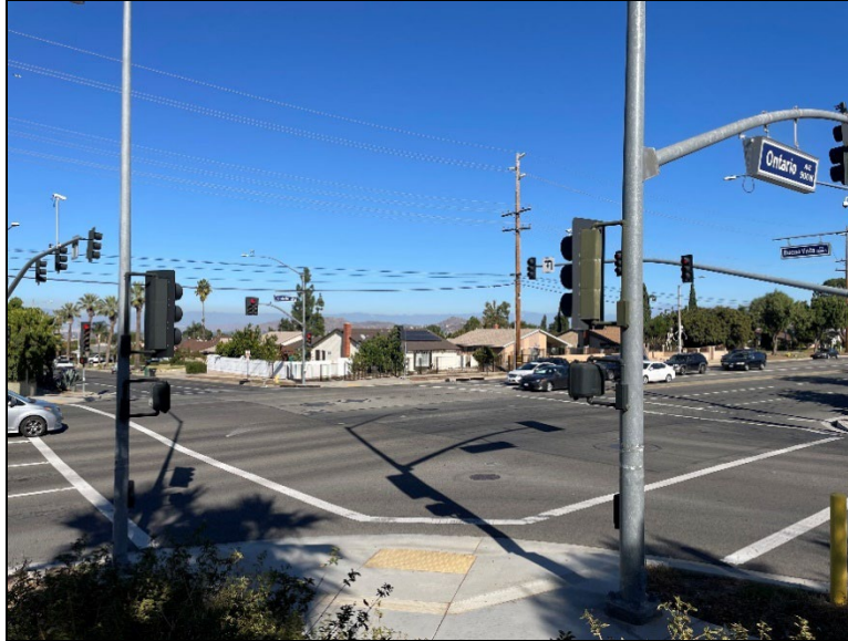
Figure 9. Buena Vista Avenue (view northeast; December 12, 2023).
