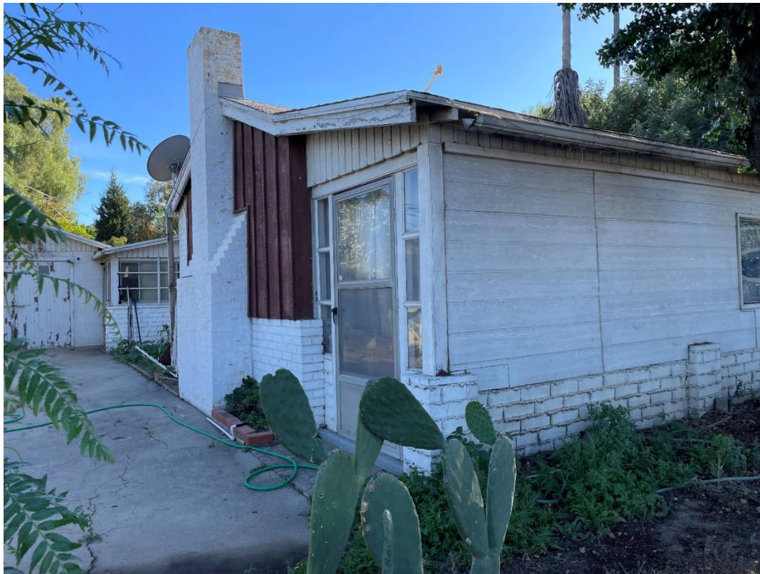
Figure 1. (View east; December 6, 2023)
