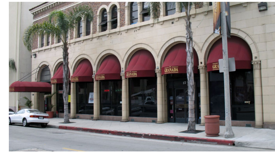
Awning placement consistent with facade design
