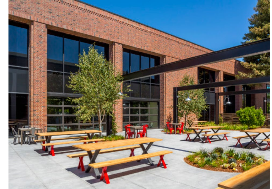
On-site courtyard with user appropriate amenities
