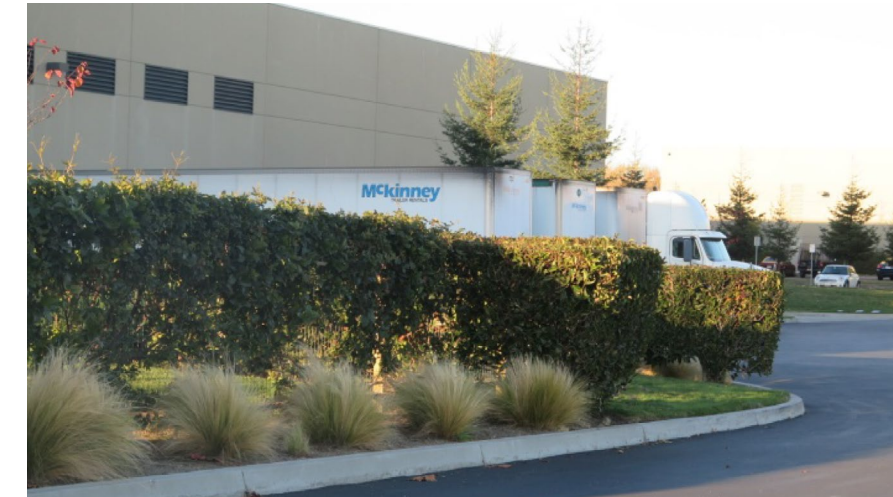
Dense plantings screen loading area
