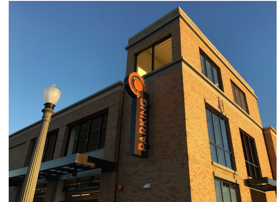
Vertical element enhance appearance of parking structure
