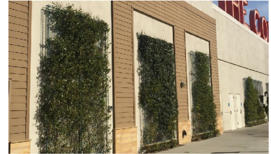
Green wall enhances otherwise blank facade.
