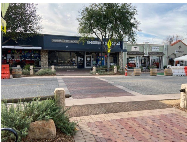
Mid-block crossing with decorative paving
