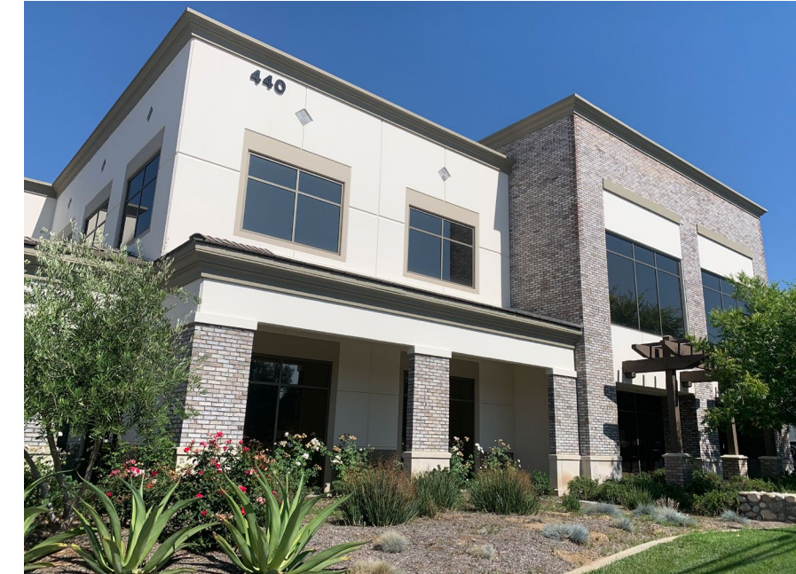
Building creates interest through vertical and horizontal offsets
