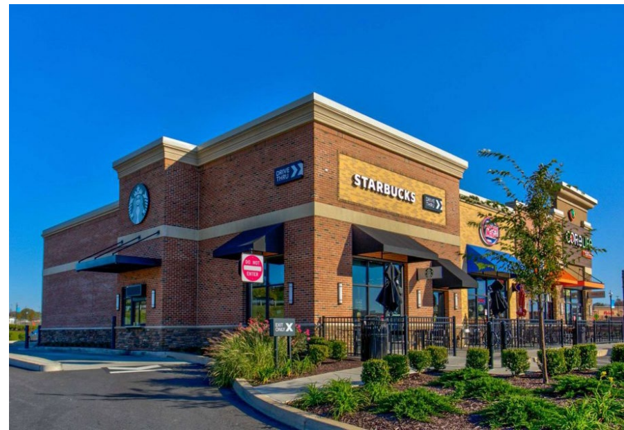
Outdoor dining area and awnings defining customer entrance
