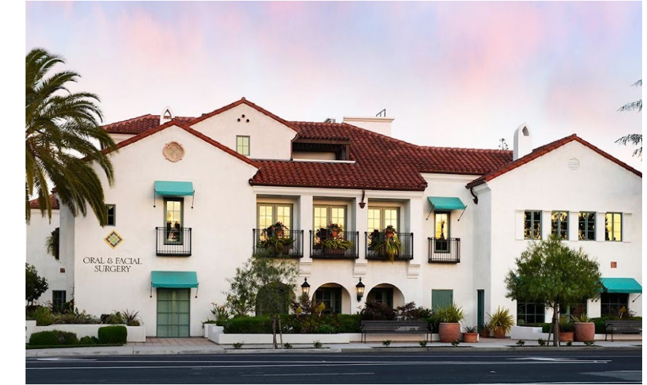
Well articulated façade with window treatments and awnings
