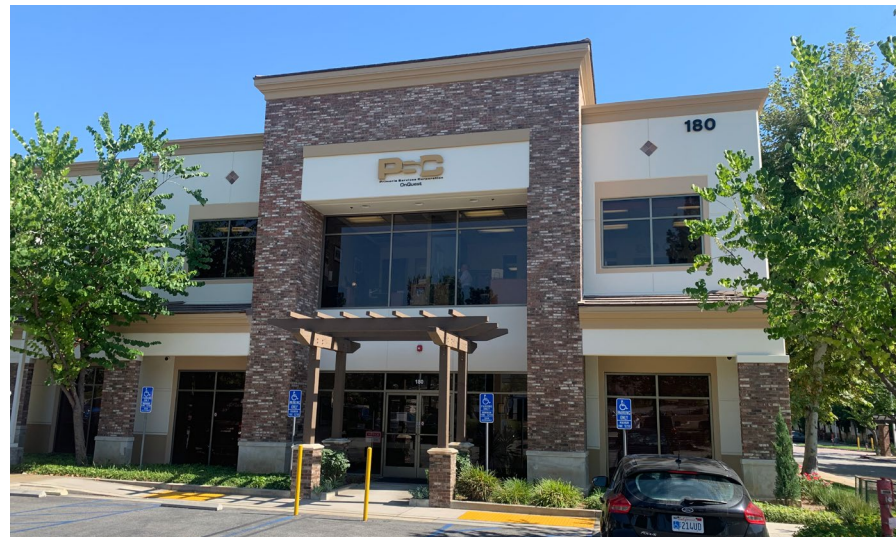
Massing accentuates main building entrance
