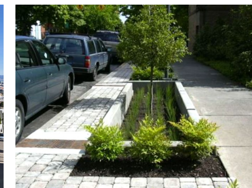
Curb-side planting with bioswale
