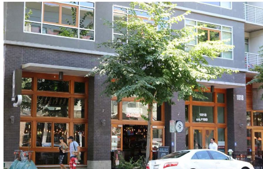
Mixed-use building showcasing harmonious high-quality materials
