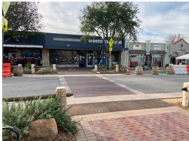
Mid-block crossing with decorative paving
