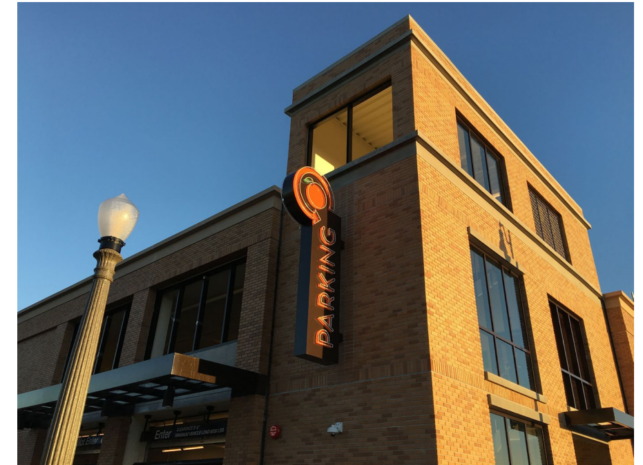
Vertical element enhance appearance of parking structure
