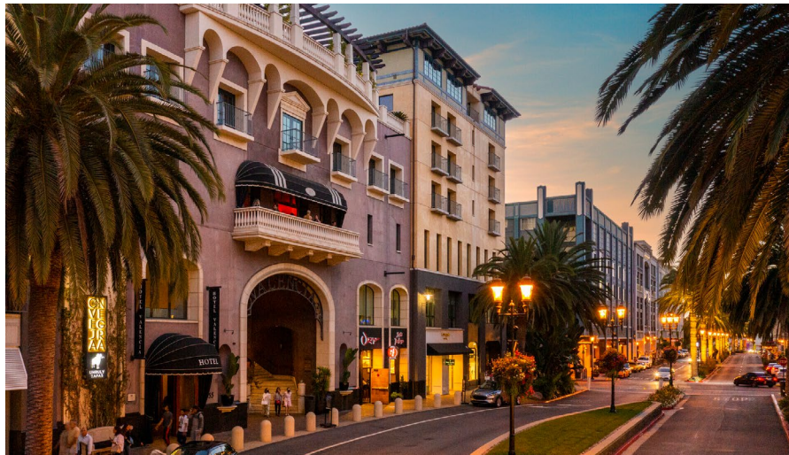
Commercial building showing modulation to give prominence to the entrance
