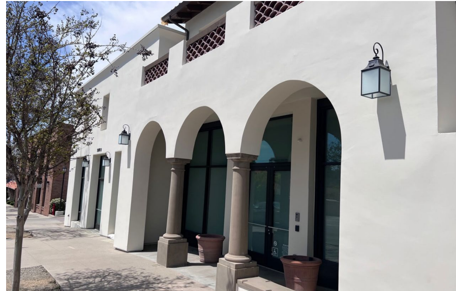
Arcade reduces visual mass and articulates facade
