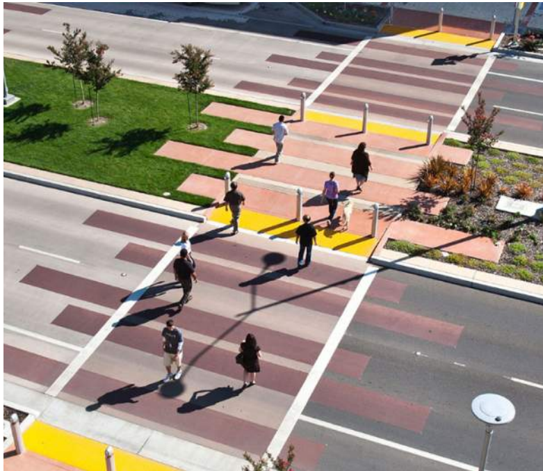
Paving graphics at pedestrian crossings (West Capitol Avenue Streetscape - Sacramento, CA) September 2024 | 6th Street Transformation | 24108
