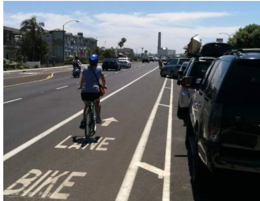
Buffered bike lane protecting cyclists from "door zone" of parked cars. (Carlsbad, CA)
