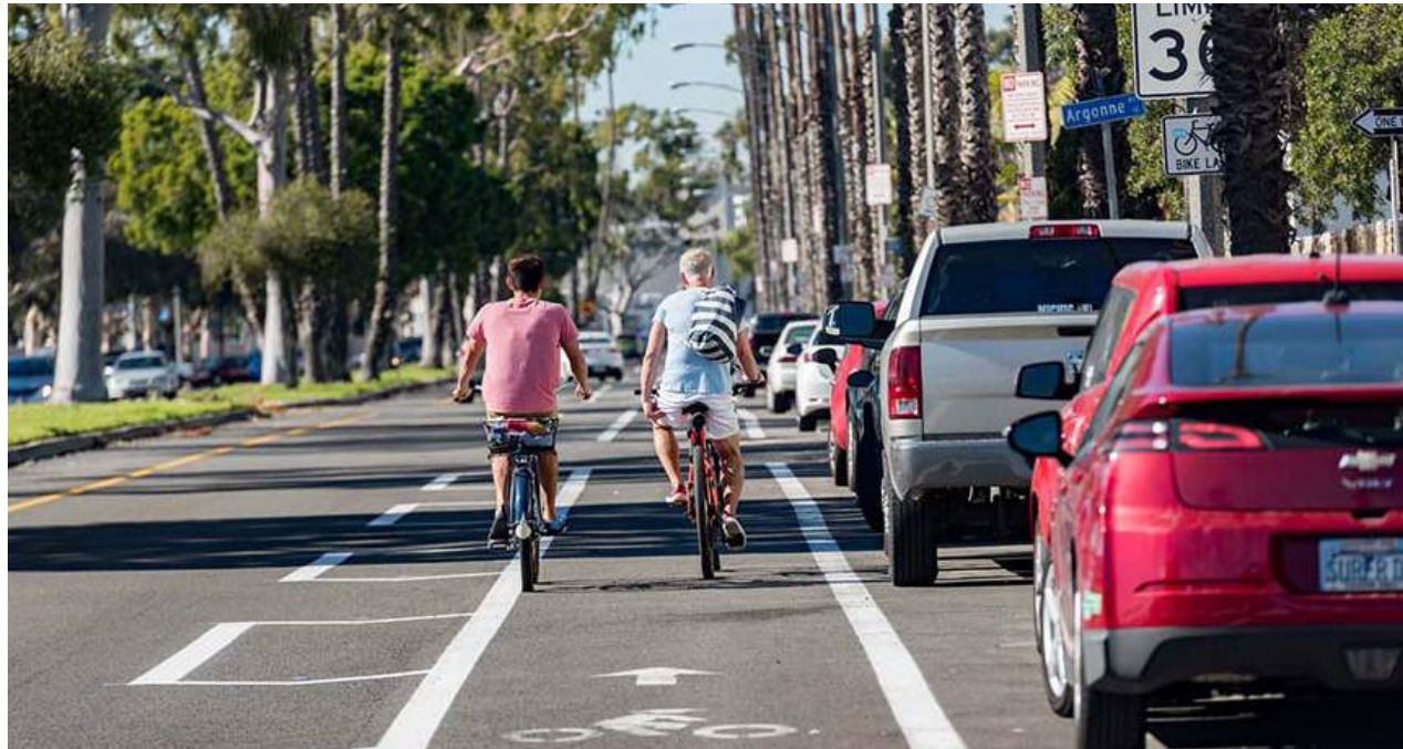
Shared travel lane for cars and bus. Buffered bike lane next to parallel parking. (Long Beach, CA)
